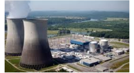
For a nuclear facility
